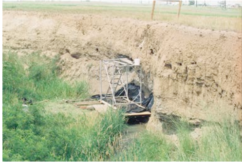
Scaffolding for excavating the hearth
