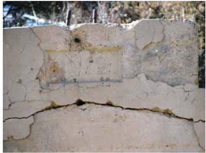
Construction date at top of jail face.
