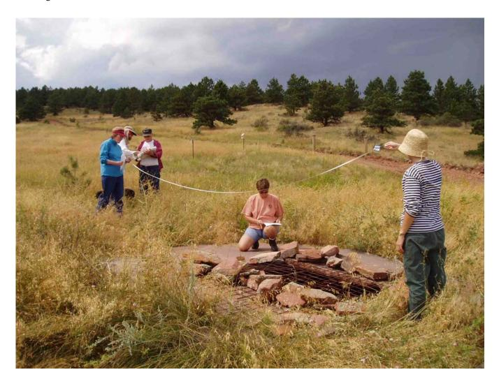
At the large cistern, left to right, Muriel Jacobs, Tom Cree, Clay Volkmann, Robyn Sloan, and Dido Clark. The cistern was dug by hand, is 9 feet in diameter, and is over 12 feet deep. It is fed by underground seepage and was reported to be used to provide water for a locomotive that transported flagstone from the quarries to the rail depot. We may excavate the bottom of the cistern. All Lyons Project photos and map by Sandy Jacobs.
